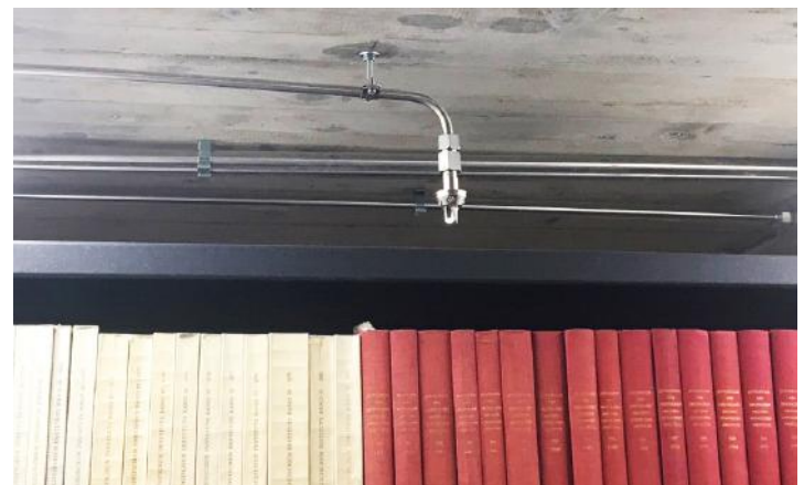
SEM-SAFE® high-pressure water mist nozzle with stainless steel Ø12 mm pipe.
