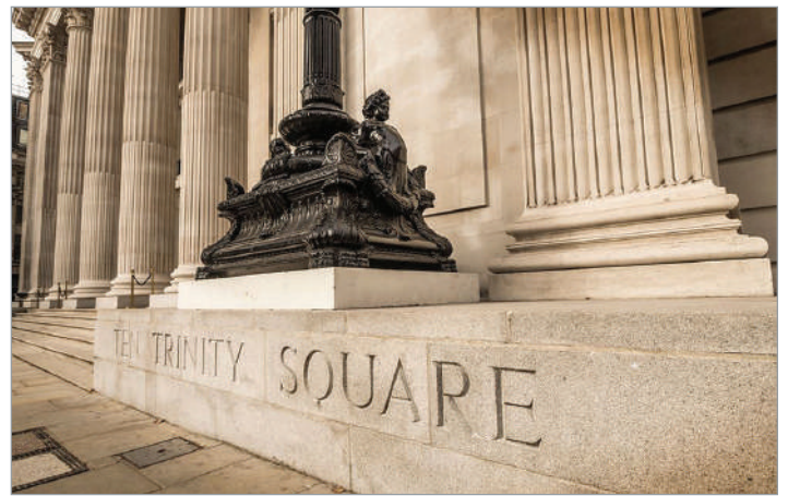
One of London's architectural icons is completely protected with SEM-SAFE® high-pressure water mist for fire fighting from Danfoss Fire Safety.
